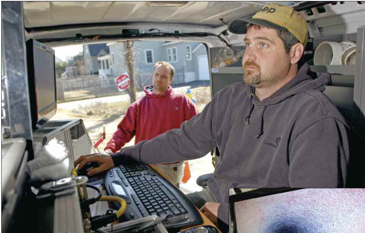
Company owner Greg Goan operates an Envirosight robotic crawler from inside a van during an inspection in Kennebunk, Maine.
